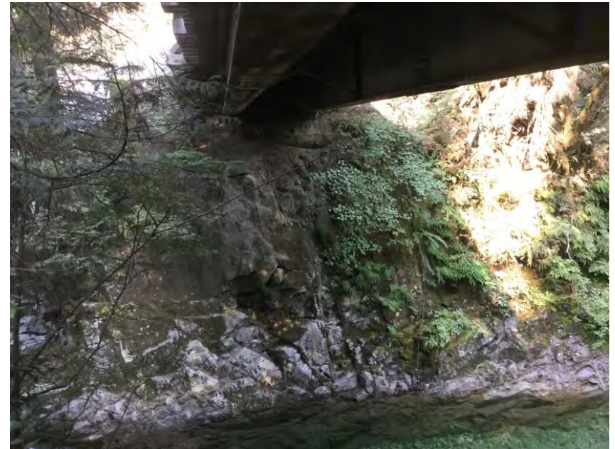
Right Bank Abutment when facing downstream
