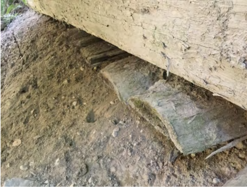
Left bank fill retaining log
