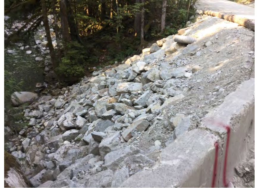
Downstream right approach riprap
